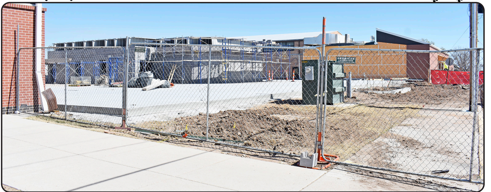
A peek inside the construction barriers and fences.
