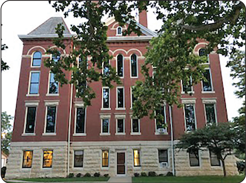
North side of the Kingman County Courthouse.
