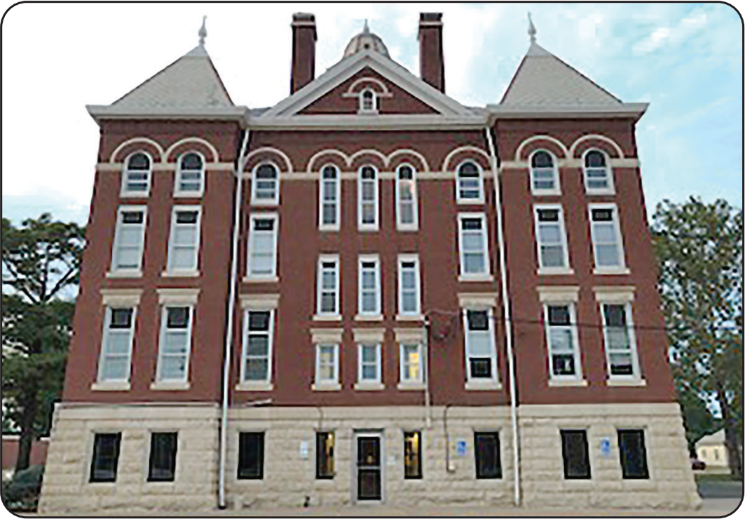
This is a photo of the south side of the Kingman County Courthouse.
