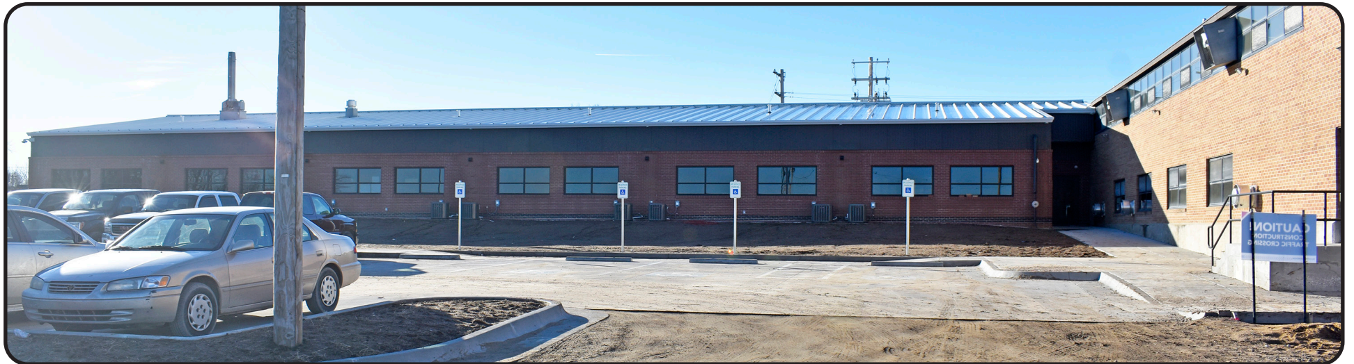
This is the north side of the new high school classrooms. they are connected to the gymnasium on the right.
