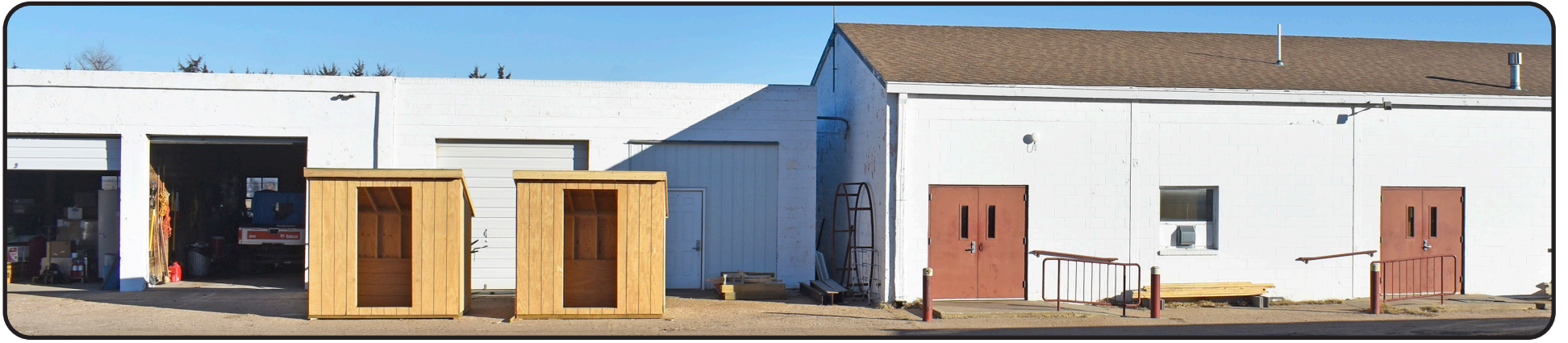
Some things don't seem to change... yet. The bus barn and the shop are still much like they have been for decades.
